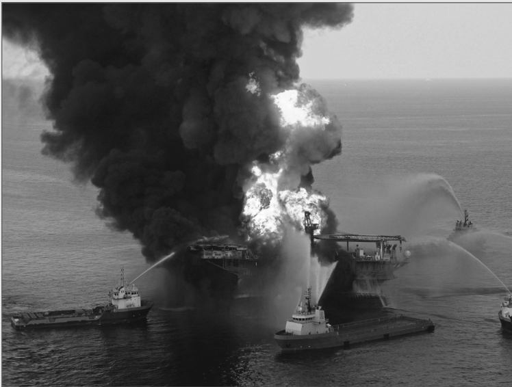
FIGURE 1.2: Deepwater Horizon Oil Rig Explosion and Fire
